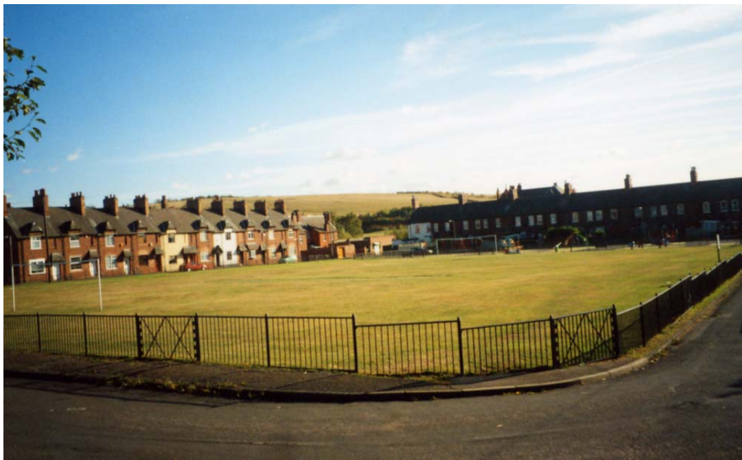
View south from Mayes Rise looking across The Square towards the former pit-head baths (These occupied the space in the centre of the photo between 2-20 The Square and 45-56 Park Road), showing the dominance of the reclaimed spoil tip and Bestwood Hotel roof upon the roofscape
