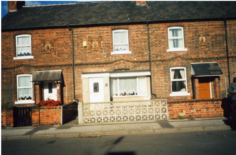
46 Park Road, showing inappropriate flat roofed front extension and replacement boundary wall, constructed during the 1980s
