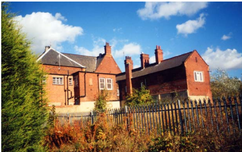
Site of former flat roofed section of Pit-head baths to the rear (south) of Bestwood Hotel. Conservation Area Enhancement schemes should significantly improve views into Bestwood Village from the Country Park
