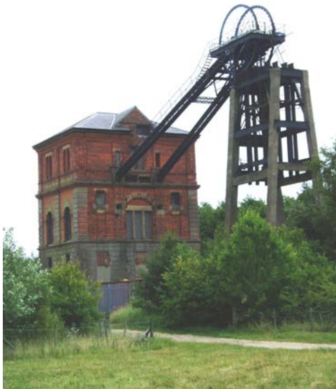
Colliery Winding Engine House, looking west (June 2004)
