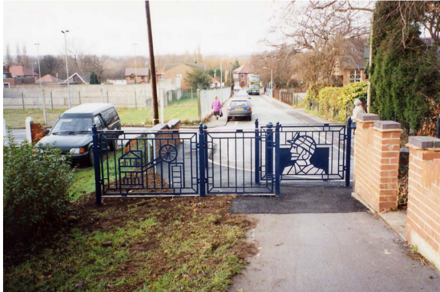
The Mount/ School Walk pedestrian railings, installed 1995
