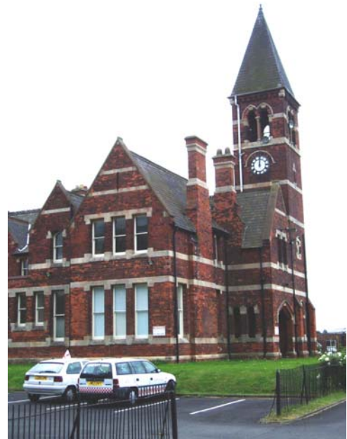
Former BICC Offices ('The Clock Tower') frontage, Park Road (June 2004)
